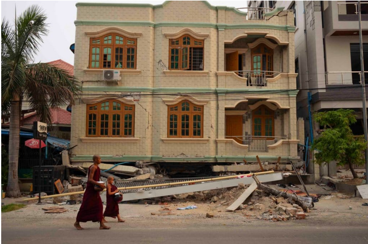
The building that collapsed in the earthquake; the first floor has been completely destroyed. Photo: Patrick Chengzhi Wang
