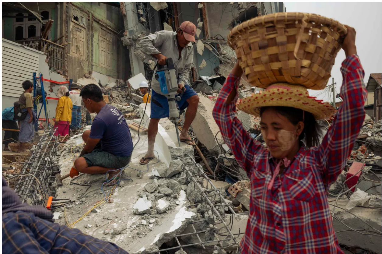
The workers are clearing the rubble. Photo: Patrick Chengzhi Wang
