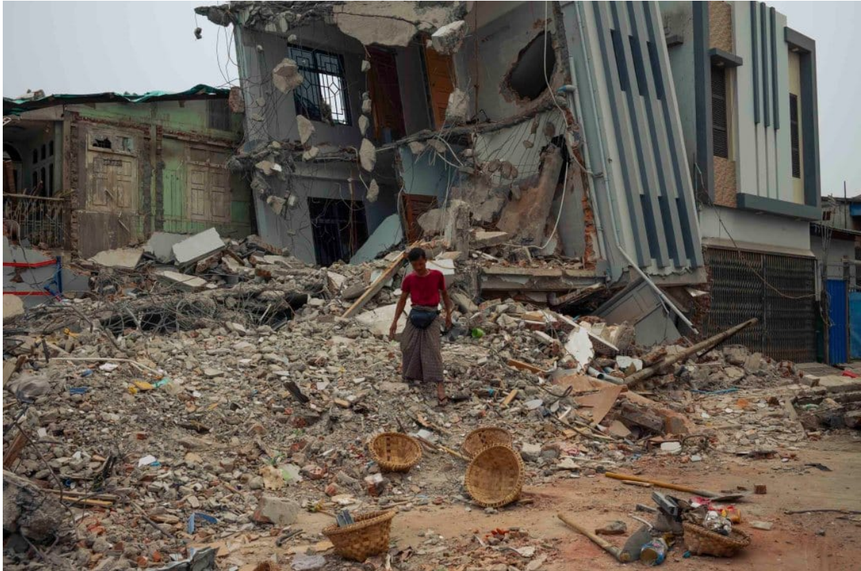
Three-story house leveled by the earthquake. No casualties. Photo: Patrick Chengzhi Wang
