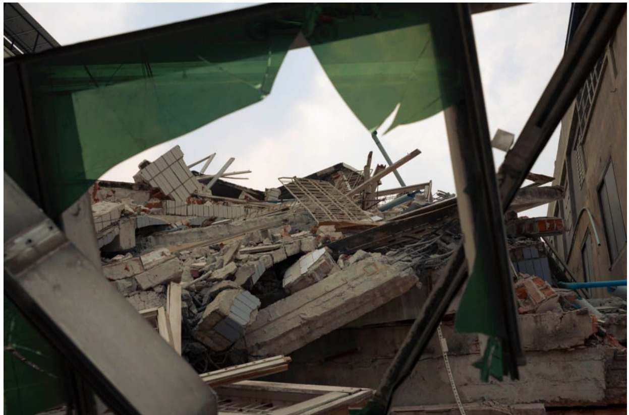
Collapsed residential structure. Photo: Patrick Chengzhi Wang
